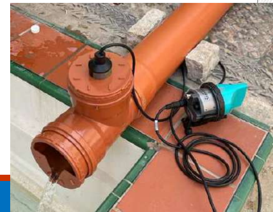
Drainage pipe. Use to transport the filtered water to the infiltration wells.
